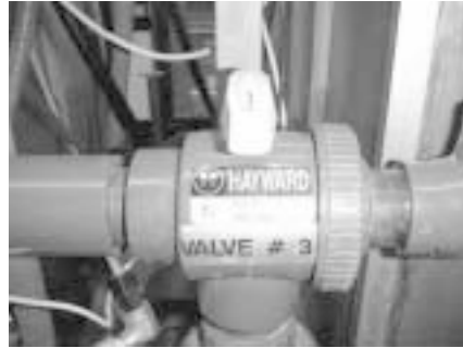
Figure 6.7—Transfer valve.
