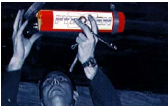
Simply installed close to the potential hazard
