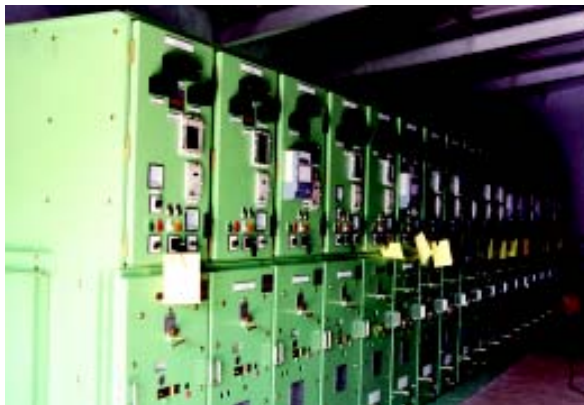
HT switchgear.
